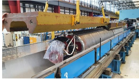
Upper alignment cradles installation
