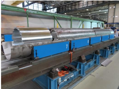
Aluminium restraint cylinders installation
