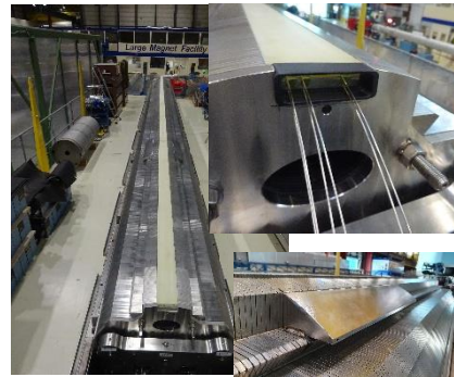
Gutter and cable puller installation Restraint alignment and welding
