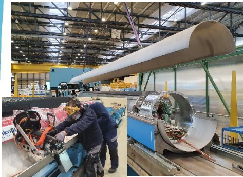
Upper shell installation after developed length machining/adjustment
