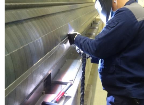
Backing strip installation and welding
