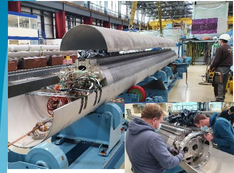
Remove upper shell Install radial restraints
