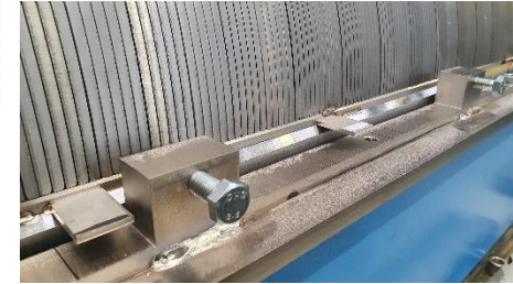
Backing strip to the shell weld and shims tack
