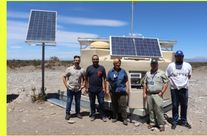
The first station of the MARTA engineering array is now installed
