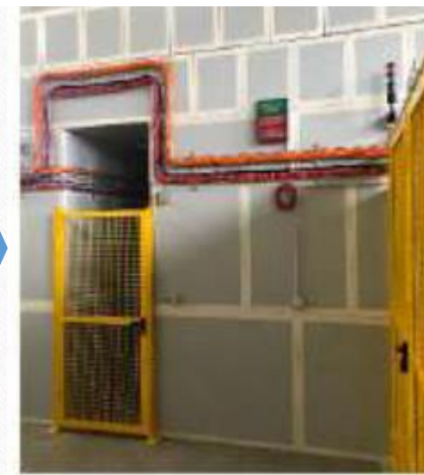
renewed RF bunker - TEX
