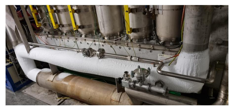
Warm-up not needed, vacuum pumping effective (DFBL warm-up requires DSL warm-up), the situation will be further monitored in the coming days. As a longer term consolidation, installation of a vacuum sensor + a complementary vacuum pumping of a secondary line
