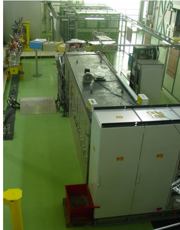
LEP-type klystron and prototype modulator under test
