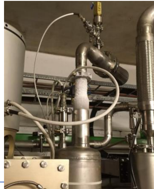
Old safety valve configuration
