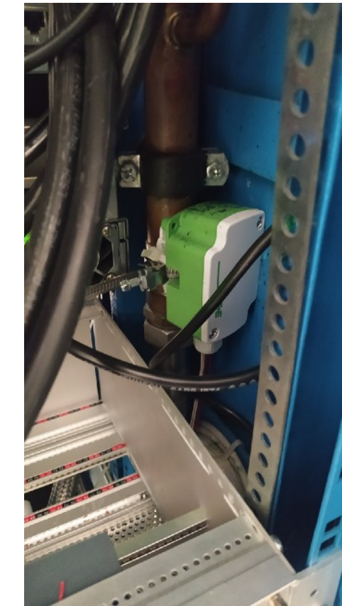
T3: temperature sensor
