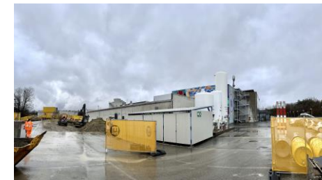
Construction of new CO 2 building at P1 (for Phase-II)
