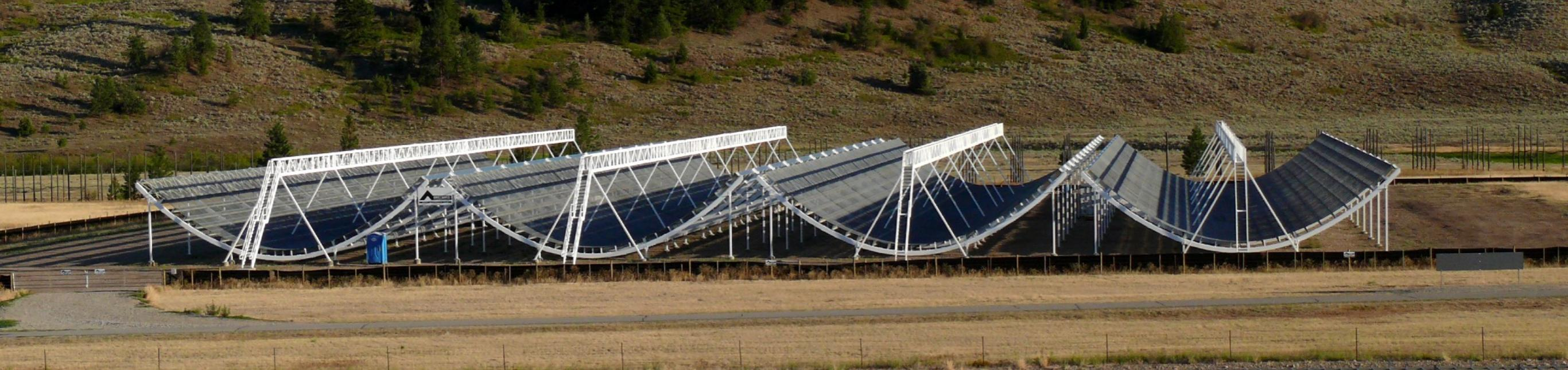
Transit radio interferometer (no moving parts)
