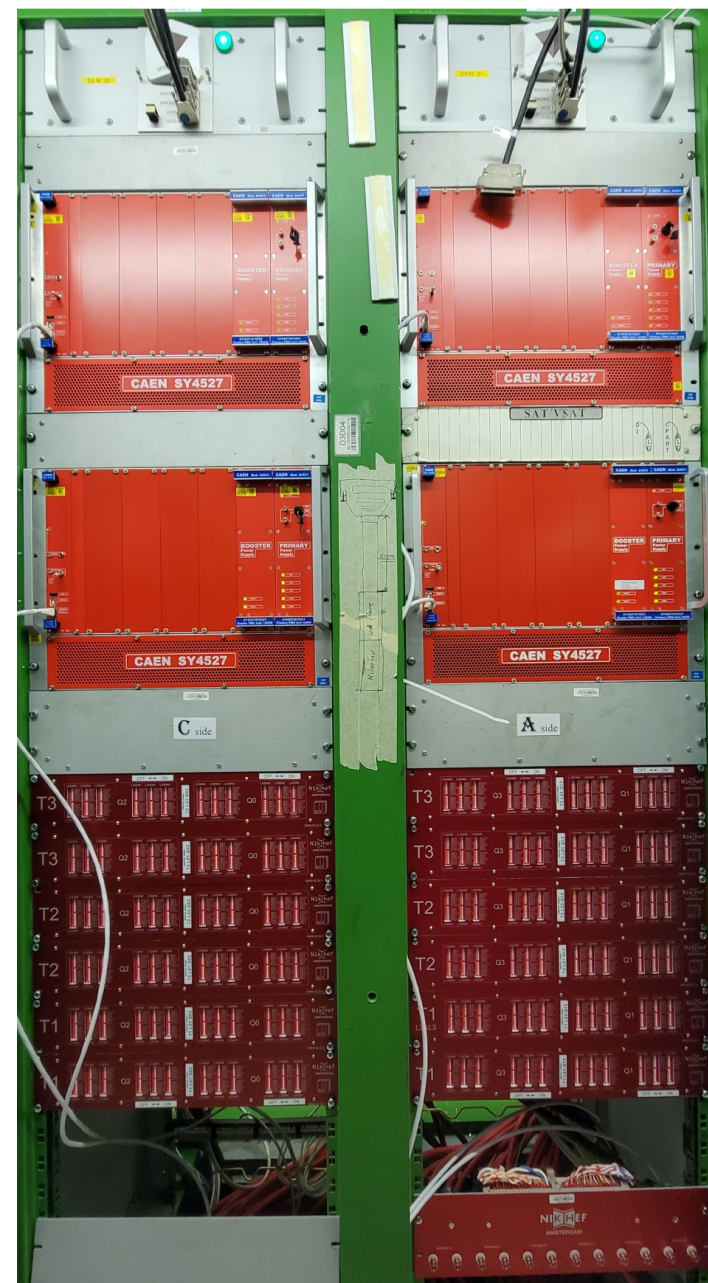
HV power supplies & patch panel
