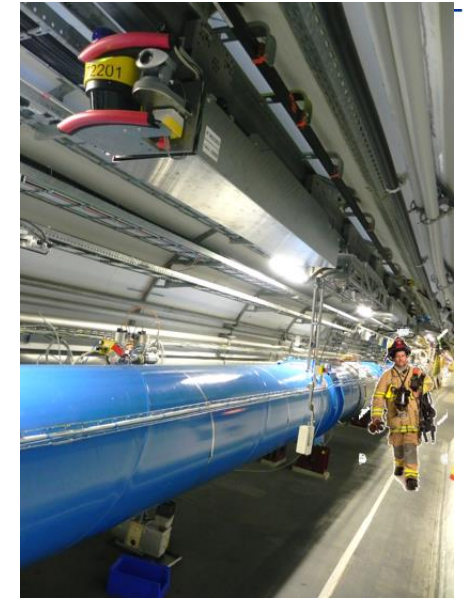
TIM escorting fire brigade personnel
