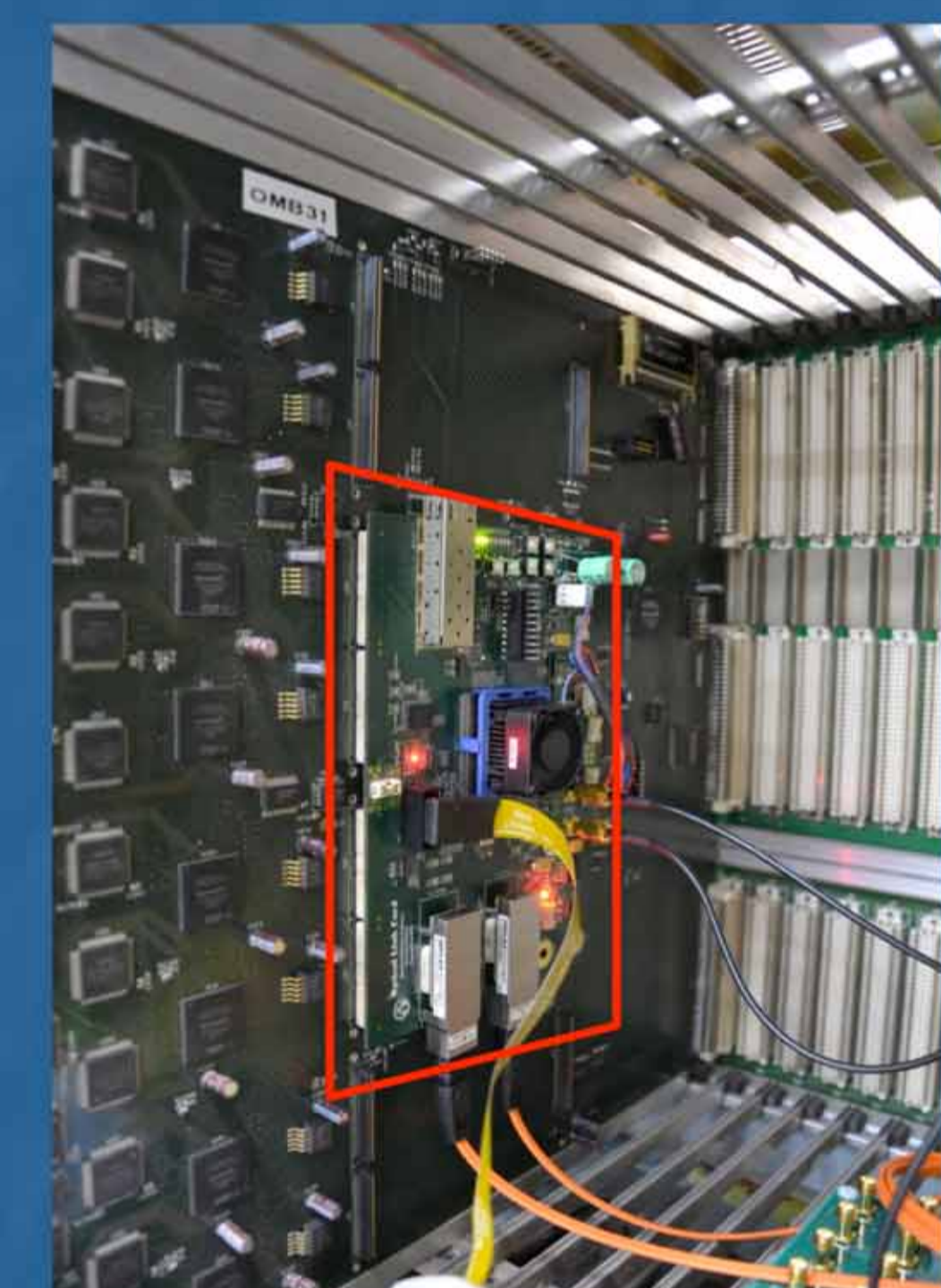
Test assembly for 12 links in bld. 175
