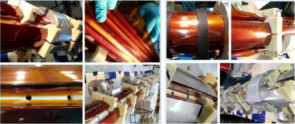
Ground insulation installation
