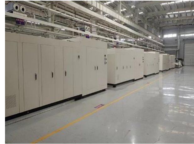
500kW Push-pull tetrode Amplifiers
