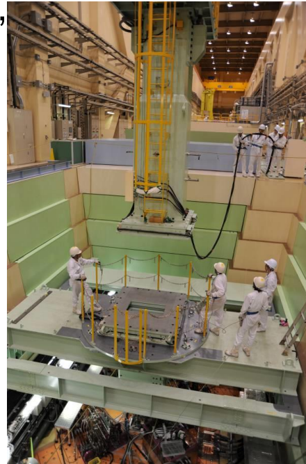
Remote controlled replacements in Hot cell
