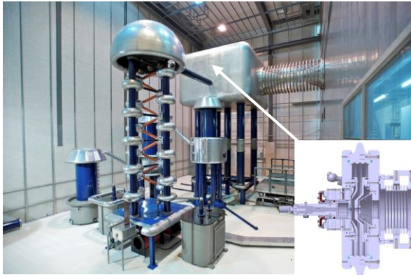
Cockcroft-Walton with 810 kV platform and acceleration tube ECR-source very reliable (>99%)
