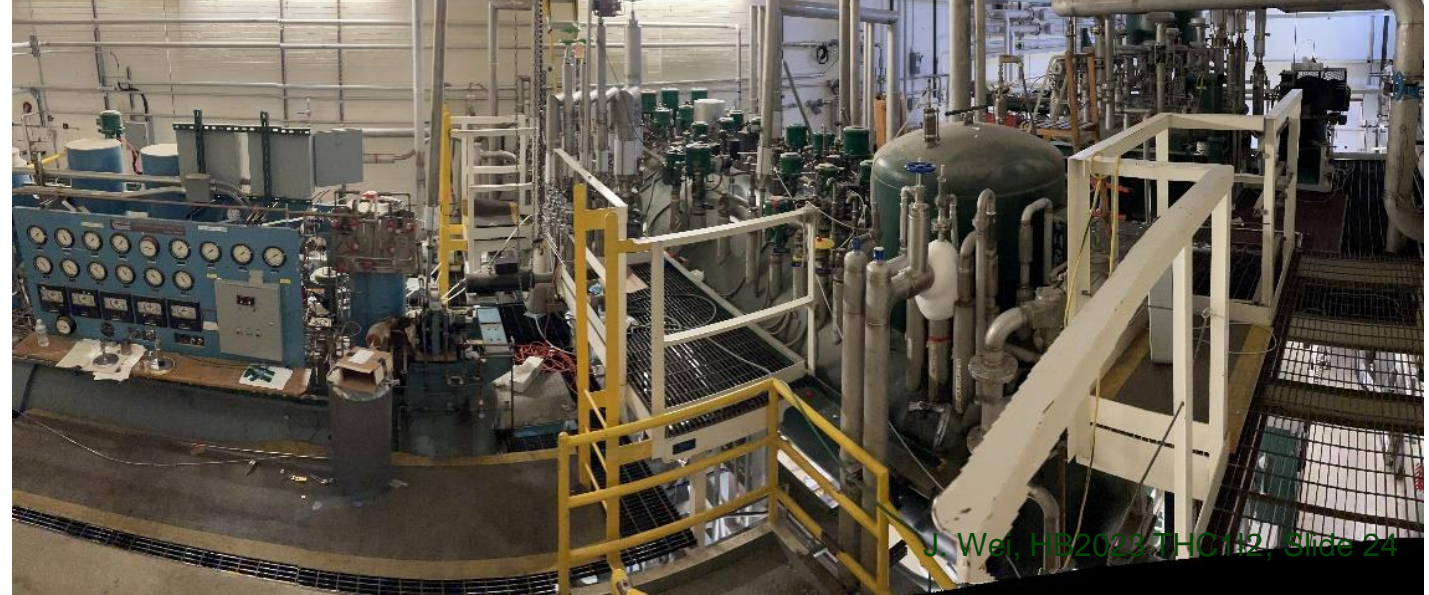
Legacy NSCL “green cold box” supporting experimental cryogenic distribution / devices
