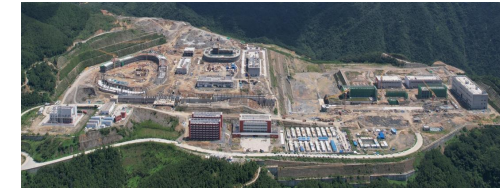
CiADS & HIAF project site
