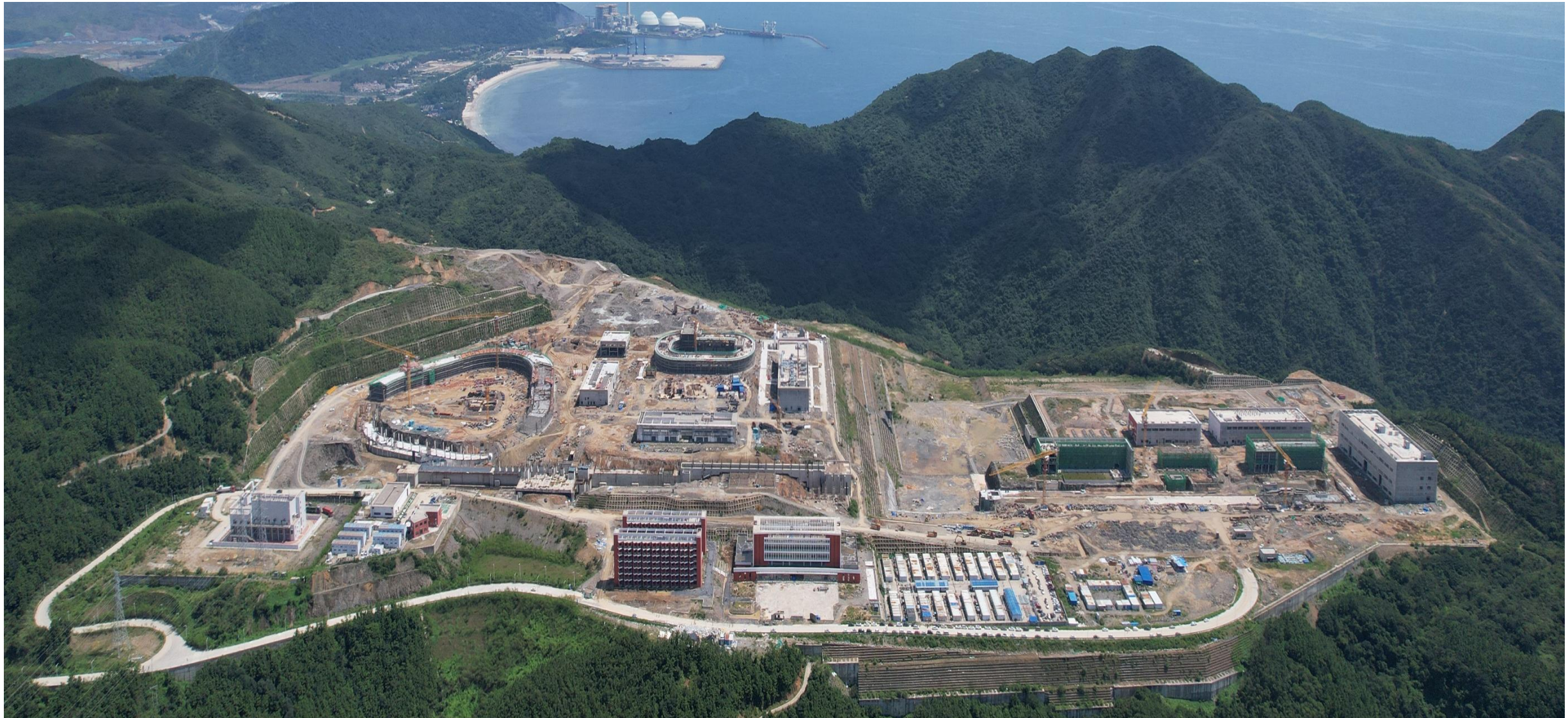
Topview of HIAF&CiADS facility construction site
