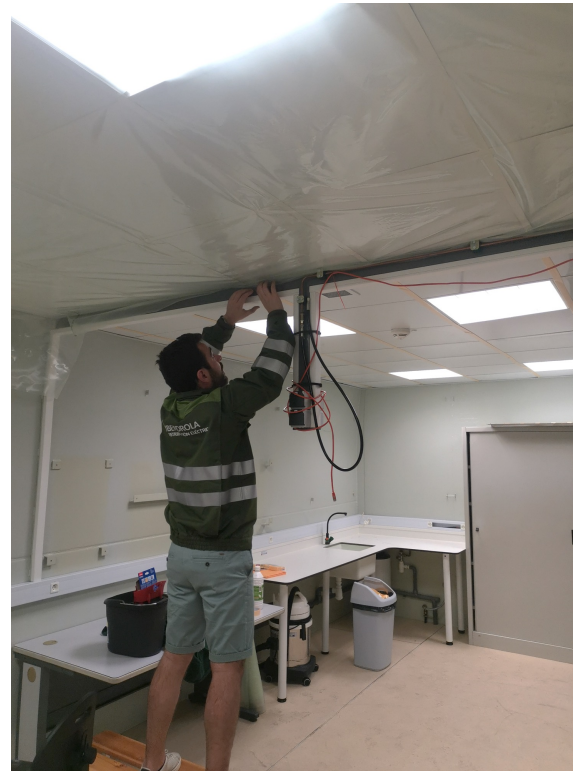
Setup of an underground clean room for detector assembly
