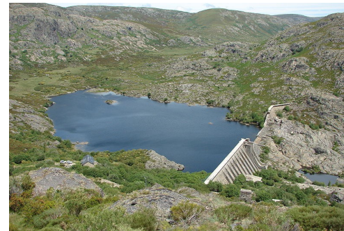
Broken dam in Vega de Tero, Spain (1959)
