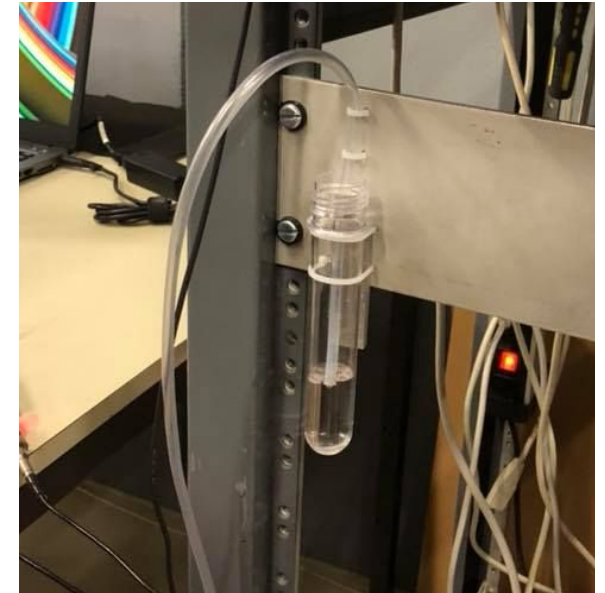
Put them under gas, fix leaks
