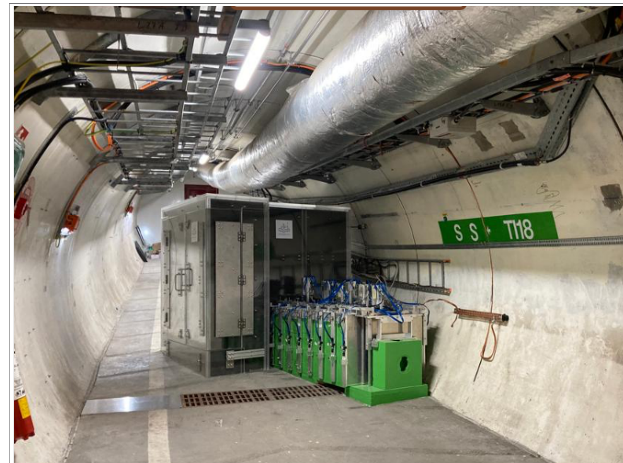
SND@LHC in the TI18 tunnel
