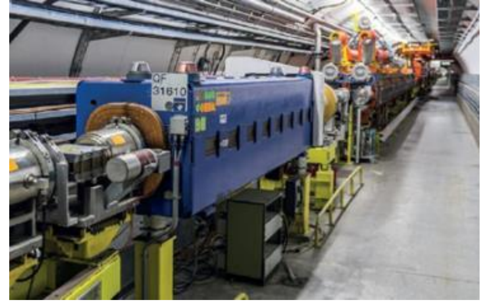
A quadrupole magnet installed in the CERN SPS
