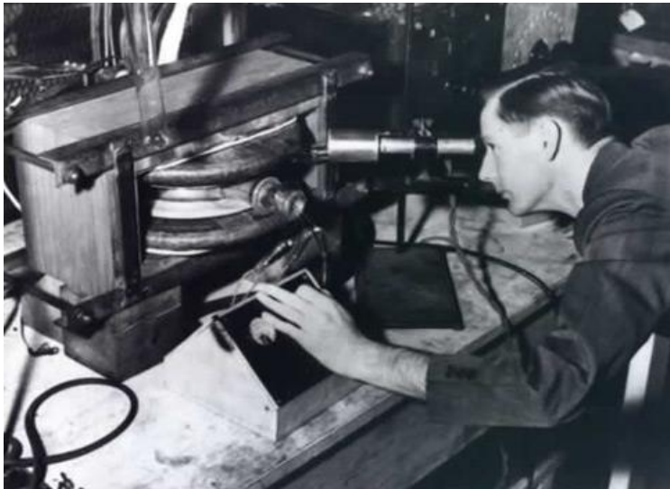
Donald Kerst with the first betatron, invented at the University of Illinois in 1940
