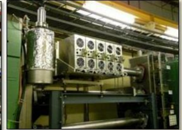
... installed in PSB ring 4
