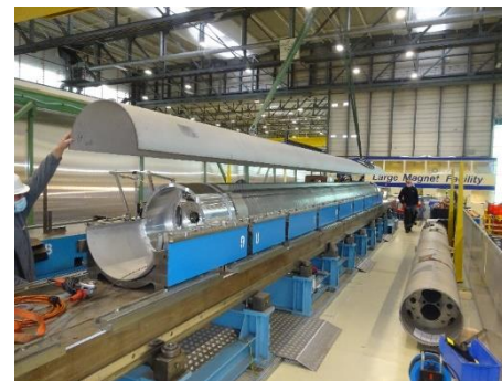
Upper shell installation on top of the magnet
