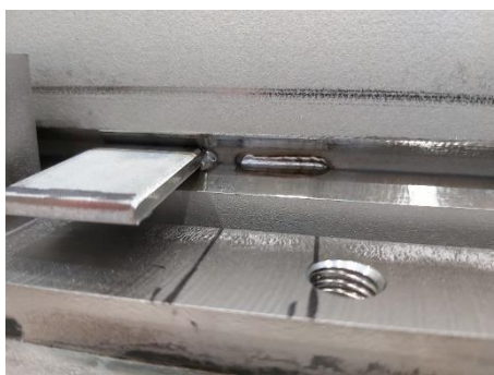
Upper shell #101 and shims tack welding to the baking strips
