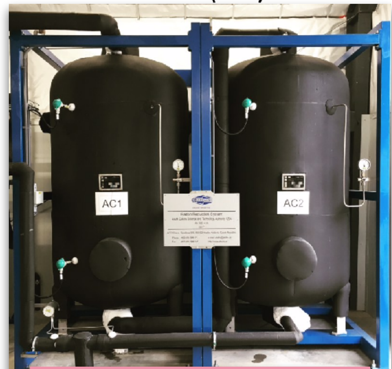
Radon reduction system at SURF
