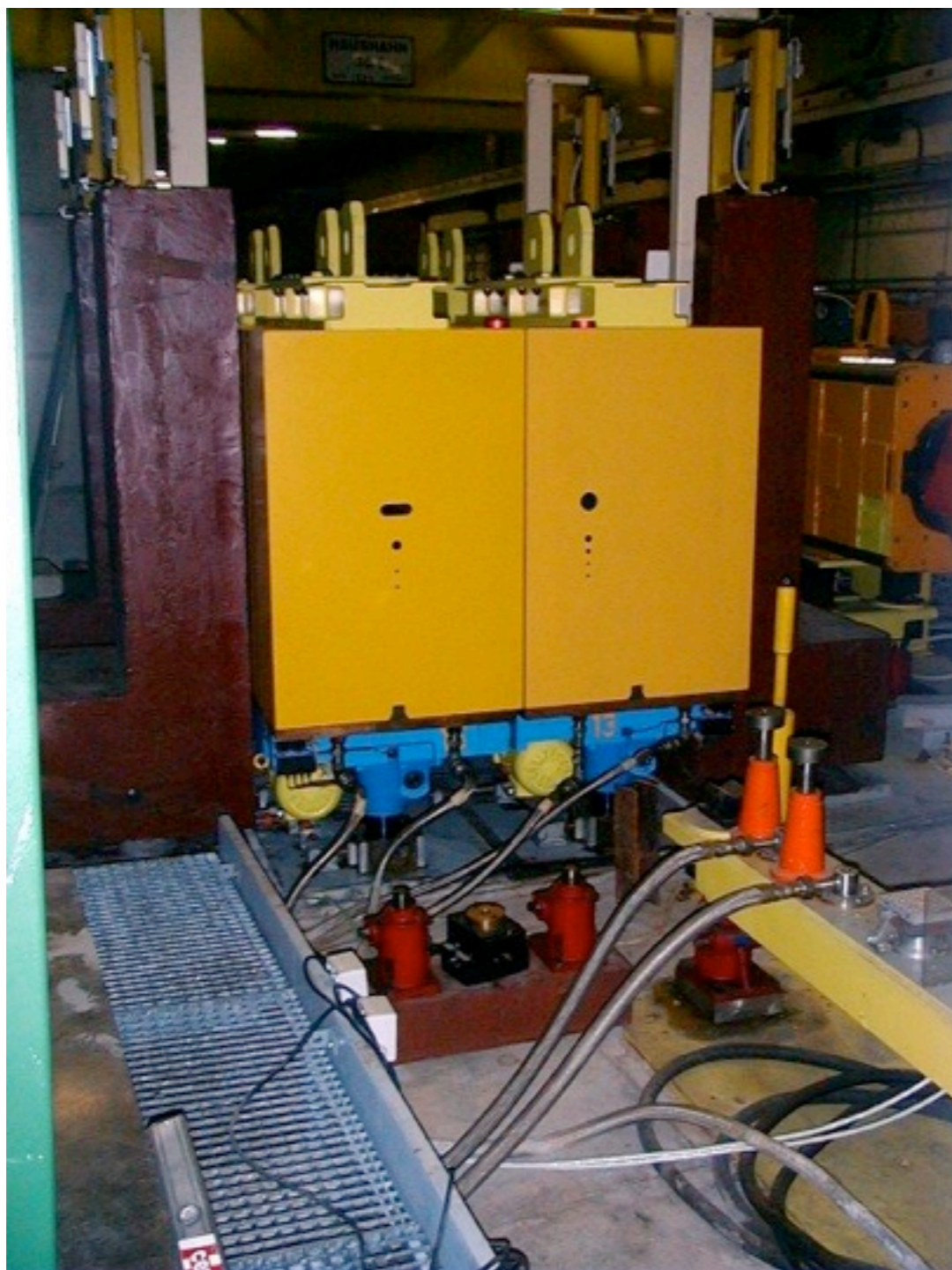
Preparation and installation of new TAX blocks for T4.
