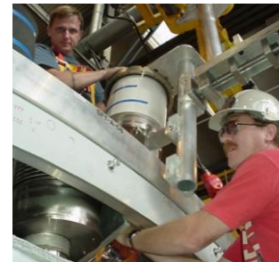
64 signal FT + 2 HV TF + Solenoid chimney
