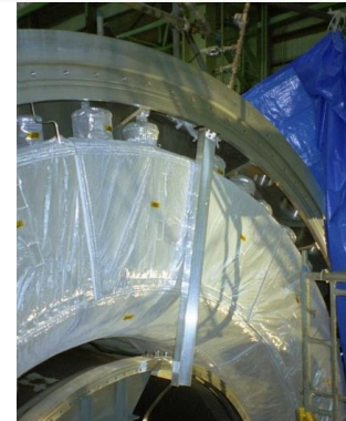
64 signal FT + 2 HV TF + Solenoid chimney
