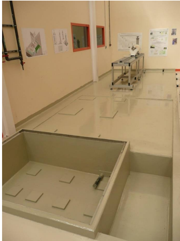
Civil engineering and floor covered with acid-resistant painting
