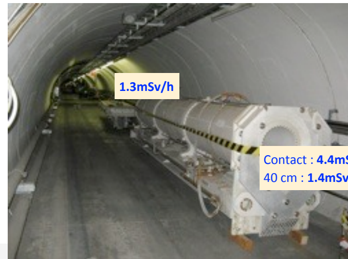
Dismantling WANF - 2010: Target & collimator
