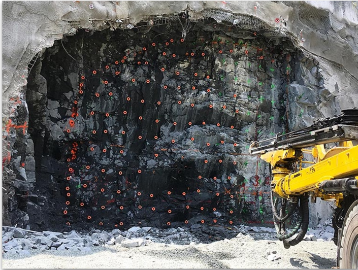
Drill and Blast
