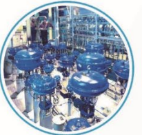
CRYOGENICS 2 new large 1.9 K helium refrigerators for HL-LHC near ATLAS and CMS will allow cryo-separation between arcs and triplet regions.
