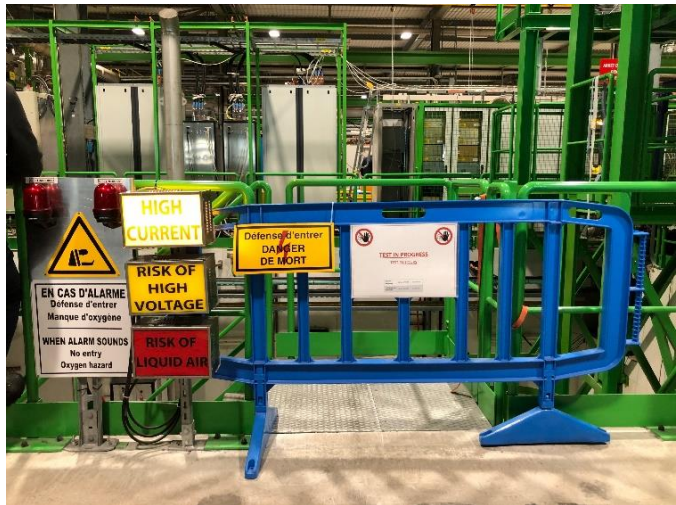
Cluster D: Gate and warning signs
