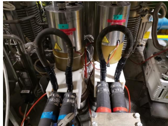
Additional insulation of live parts
