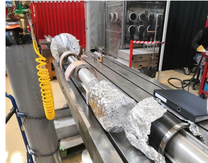
Busbar line being manufactured in main workshop
