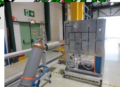
Pressure test of cooling tubes
