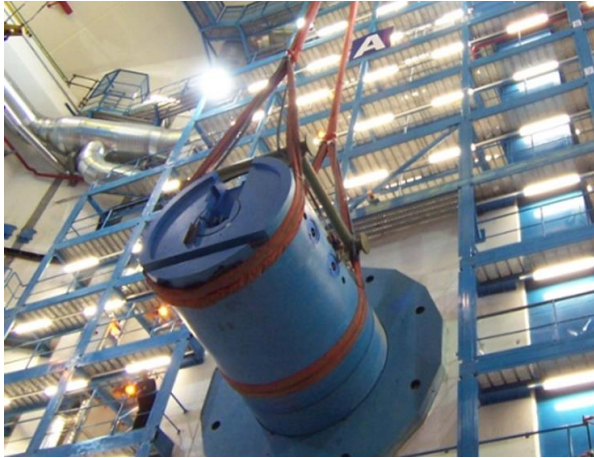
ATLAS Forward Shielding (here Monoblock TX1S insertion into Fixtube)
