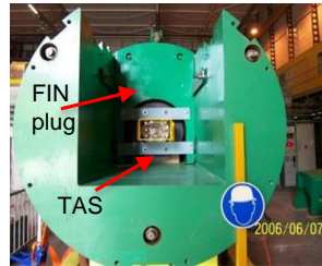
ATLAS Forward Shielding (here Monoblock TX1S insertion into Fixtube)
