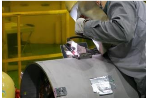
Welding of alignment markers
