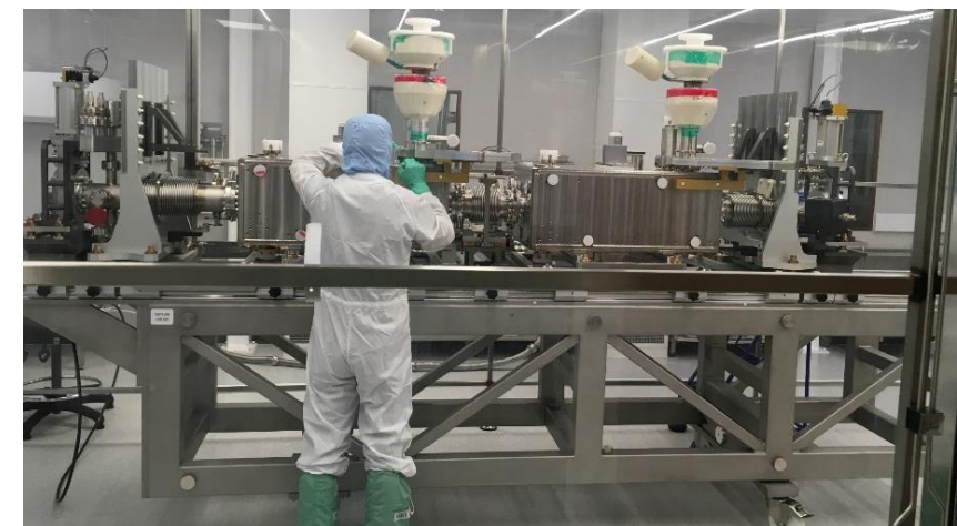
FPC installed to cavity x2 (Cleanroom ISO4)
