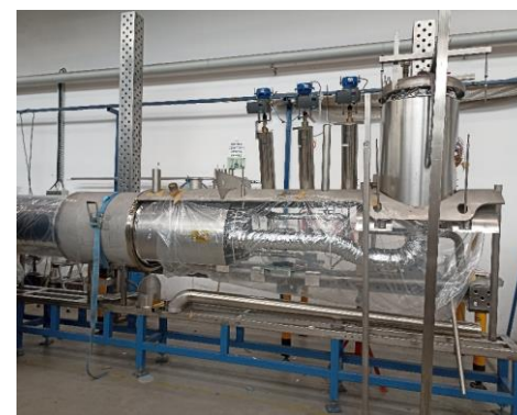
Assembly of the return module at Kriosystem.
