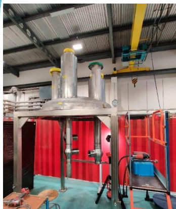
CCU box being refurbished
