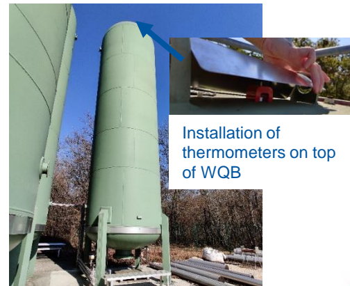
WQB connected to SM18 cryo infrastructure
