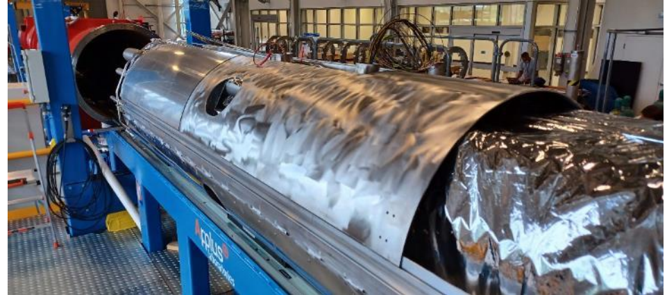
Installation of thermal shield after cold mass MLI installation
