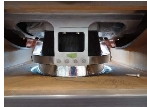
Thermal shield support installed
