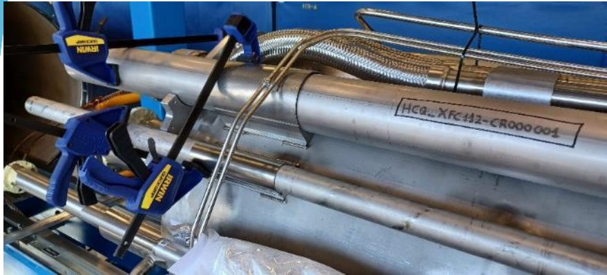
Installation of piping
