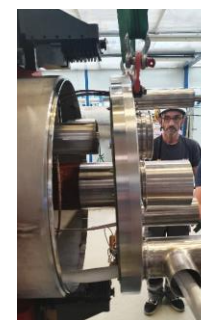
End covers alignment and welding
