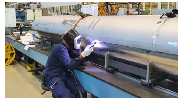
Shell tack welding to the backing strips
