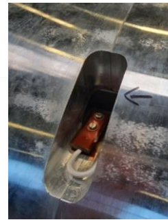
Thermometers installation
