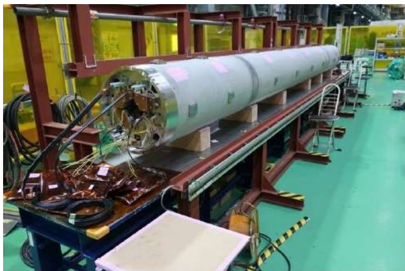
Shell Welding completed
