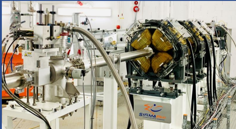
R&D beamline, Manchester Hospital (UK)
