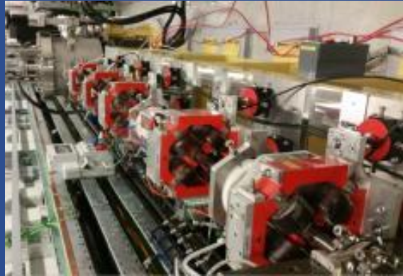
Quadrupoles – Elettra synchrotron (Trieste, Italy)
