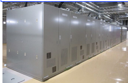
New main magnet PS for high repetition rate
