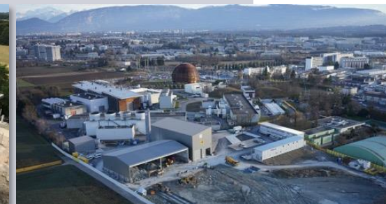
P1 - 60% of excavated material treated on site - topsoil reclaimed
