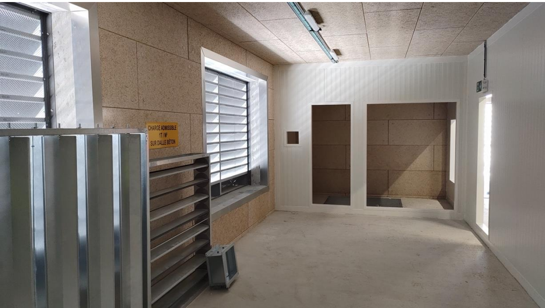
CV room (plenum installation)
