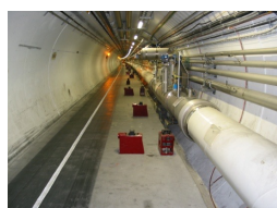
Cryogenic distribution line
