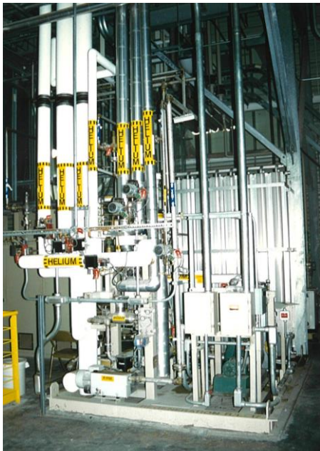
Regeneration System for the 80 K and 20 K adsorbers at 4.5K cold box. NOTE: Picture from SSCL
