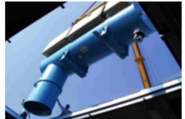
2.4 kW 1.8 K Refrigerator for LHC
