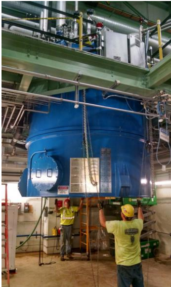
Figure 6: Removal of coldbox heat exchanger E3120
