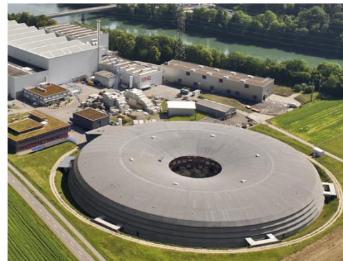
SLS, 2001, Switzerland: 2.4 GeV, 288 m ring, 16 beamlines, to be upgraded to DLSR during 2023-2025
