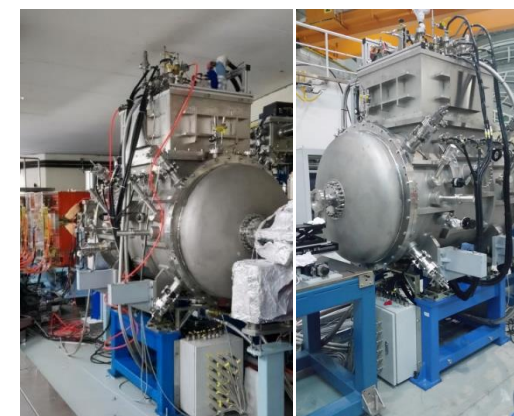
SCU installed in SSRF storage ring
