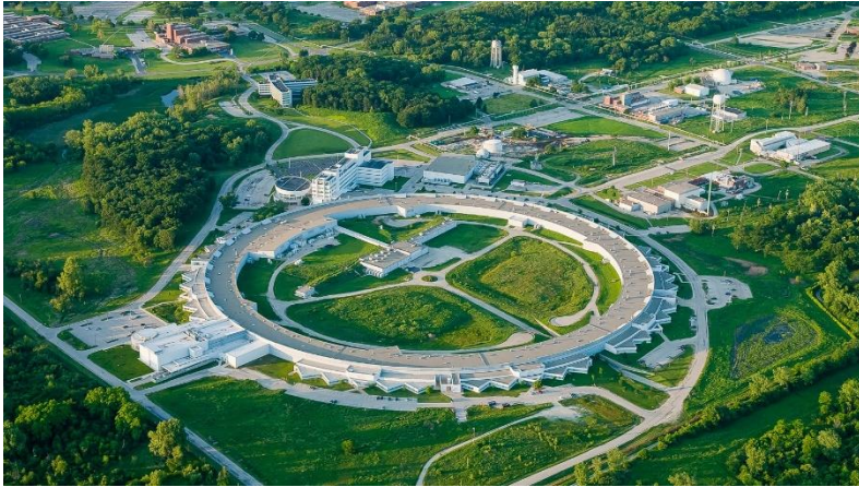
APS, 1995, USA: 7 GeV, 1104 m ring, 35 beamlines; to be upgraded to DLSR during 2023-2024
