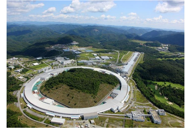
SPRING8, 1999, Japan: 8 GeV, 1436 m ring, 48 beamlines
